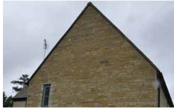
Steeply pitched roof with no overhang, Bletchington
