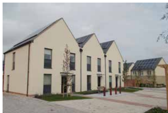
A shared surface street - NW Bicester
