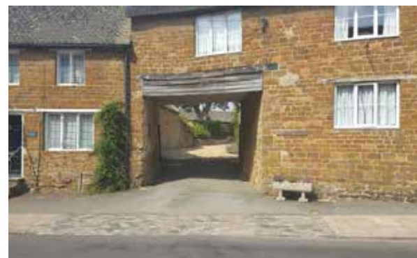
Rear parking accessed through carriage arch, High Street, Adderbury
