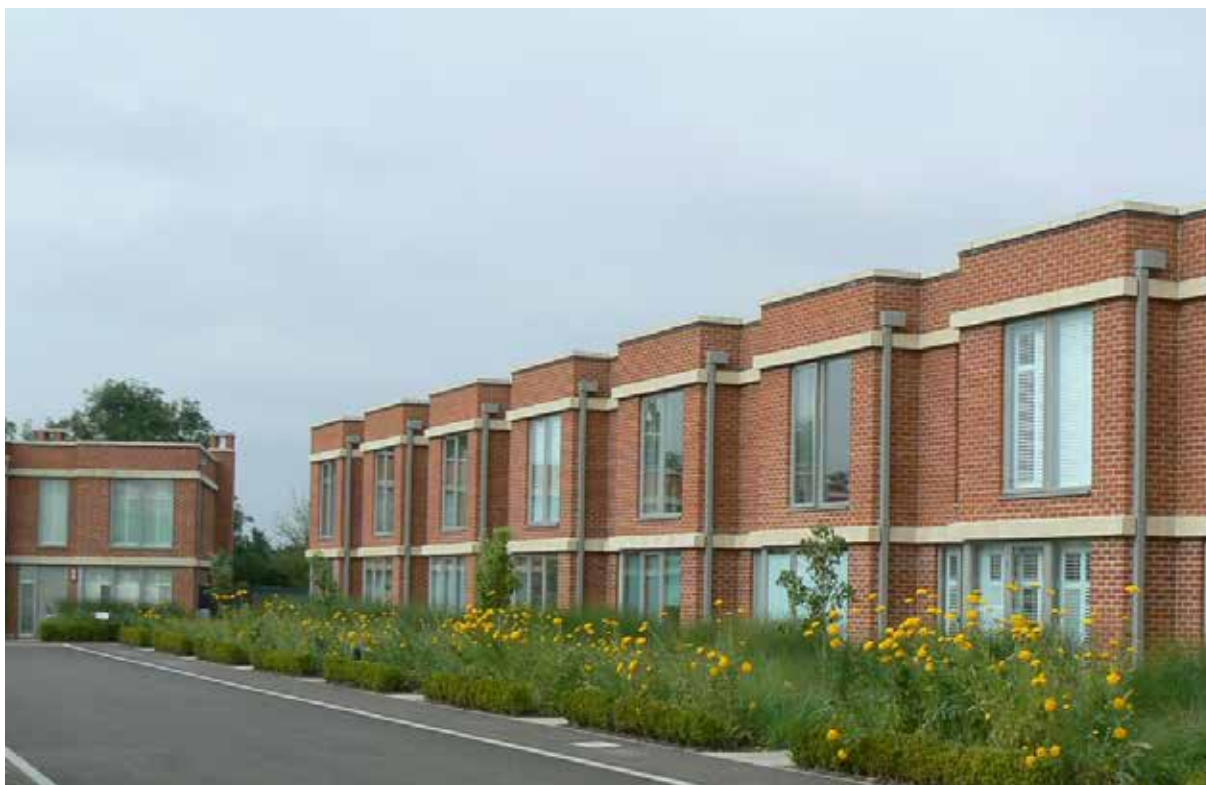
Consistent street frontage, Bicester
