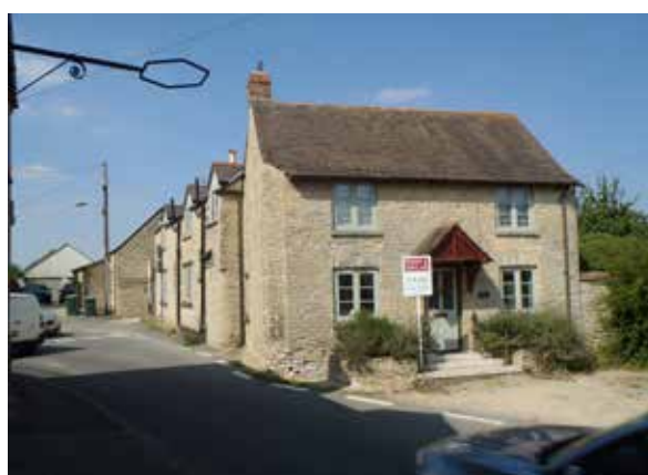
Corner of building juts out into the road, creating a natural pinch point forcing cars to give way to oncoming traffic, Islip
